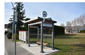
Concrete pads for transit shelters installed
