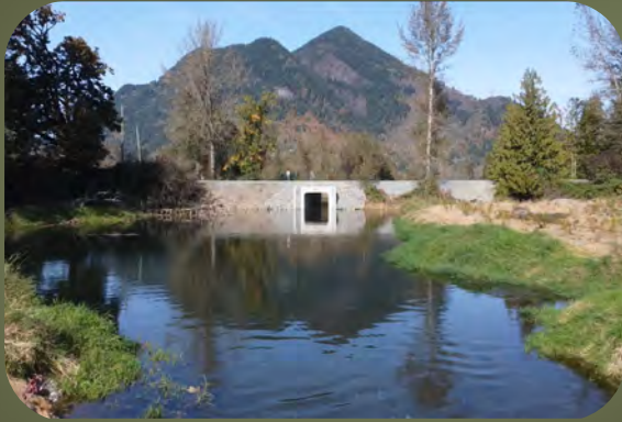
New Chaplin Road box culvert in the Maria Slough.
