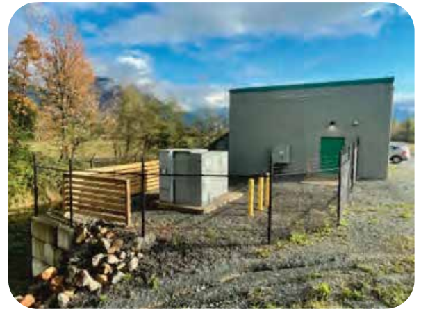
Hammersley Drainage Pump Station.
